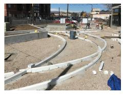
FortaCast® installed directly on paver bedding. FortaCast® can also be installed in existing concrete or bituminous paving using standard paving techniques.
