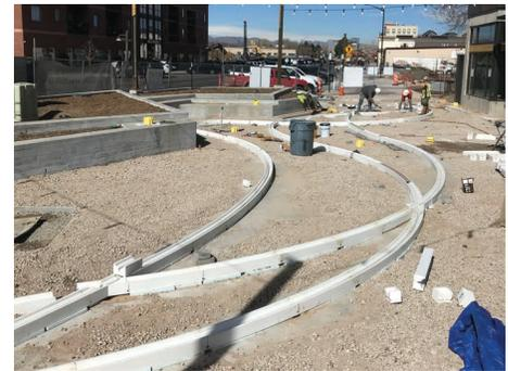
FortaCast® installed directly on paver bedding. FortaCast® can also be installed in existing concrete or bituminous paving using standard paving techniques.
